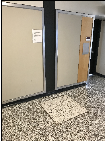
Figure 1 - Example Crawlspace Access Point (Block B)
