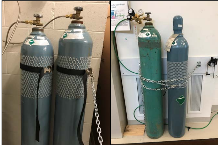
Figure 9 – Securing compressed gas cylinders.
