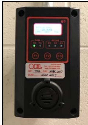
Figure 16 - Example of an oxygen sensor
