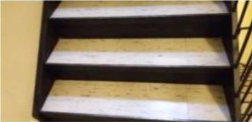
Photo 1: View of asbestos-containing vinyl floor tiles (9"x9"-White and Black) observed to be in good condition in C207C.
