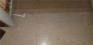
Photo 2: View of asbestos-containing vinyl floor tiles (12"x12"-Cream and Brown Coloured) observed to be in good condition in Room W0041.
