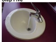
**Run Cold Water 5 Minutes** to remove residue bleach solution.
