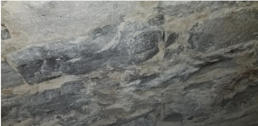
Photo 4: View of non-asbestos containing foundation block mortar observed in the basement level of the subject building.
