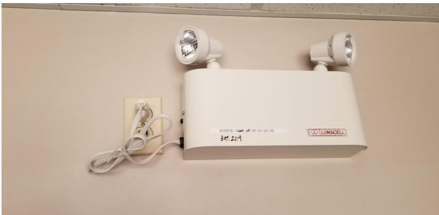
Photo 6: View of lead acid battery pack observed to be in good condition in Room 301.
