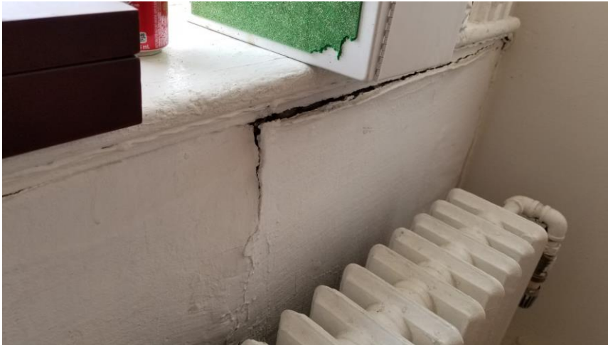
Photo 4: View of non-asbestos containing wall plaster observed in Room 310.
