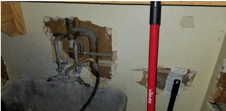
Photo 5: View of asbestos-containing drywall joint compound observed to be in poor condition in Room 314. Repaired September 2020.
