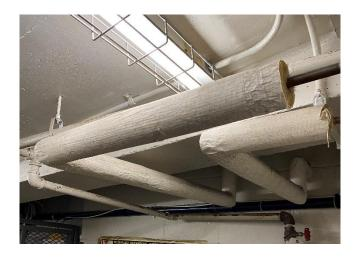
Photo 1: View of fiberglass pipe insulation observed throughout the subject building.
