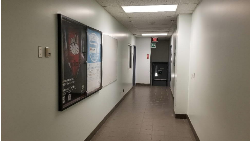
Photo 1: Representative view of the interior finishes observed in the subject building.
