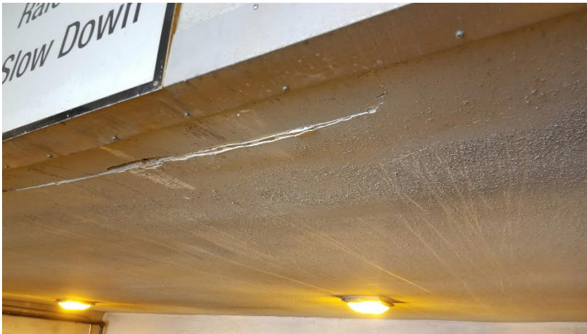
Photo 14: Representative view of the non-asbestos cementitious coating observed in Room 007.
