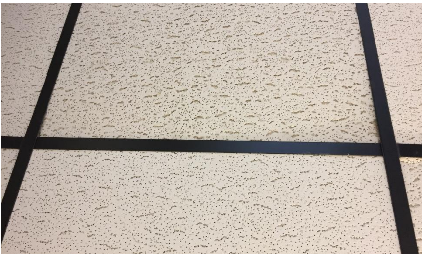
Photo 3: View of the non-asbestos containing ceiling tiles identified throughout the subject building.
