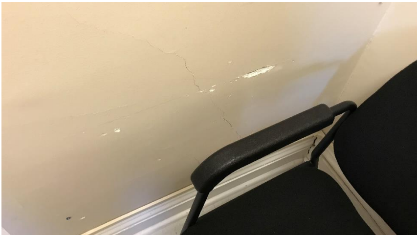
Photo 2: View of the non-asbestos containing wall plaster observed throughout the subject building.
