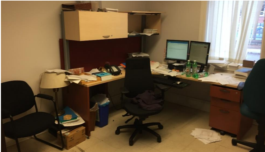
Photo 1: View of the interior finishes observed throughout the subject building.
