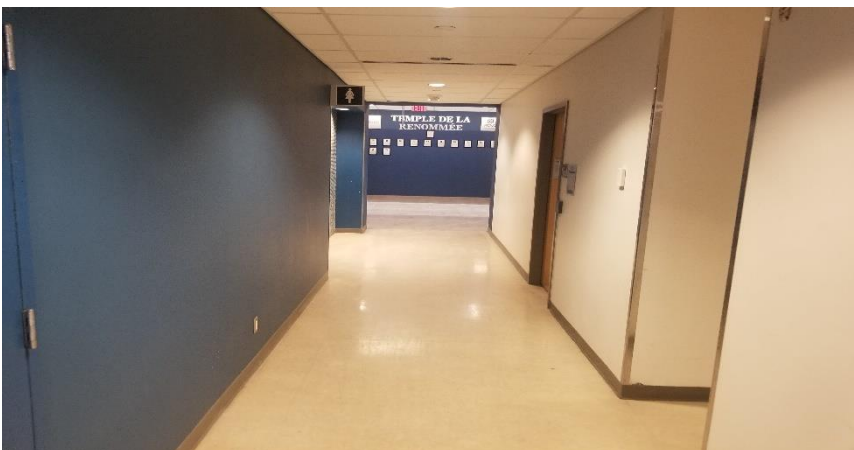
Photo 3: View of typical hallway finishes with lead-acid batteries present in emergency lights.
