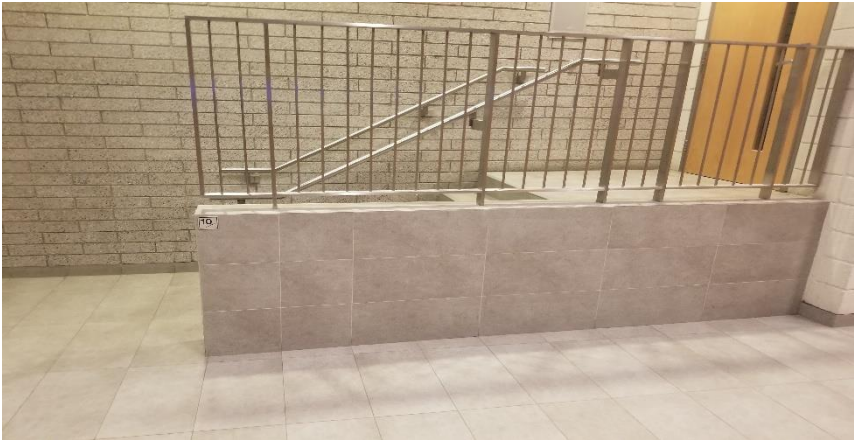
Photo 4: Typical silica containing brick, mortar, concrete and ceramic tile finishes.
