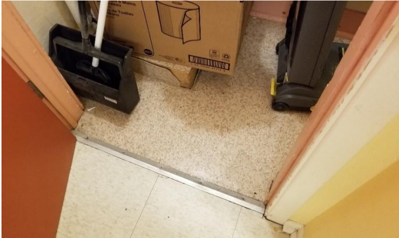
Photo 4: View of non-asbestos vinyl sheet flooring (Grey and White) and non-asbestos 12"x12" vinyl floor tiles (White w/ Grey Flakes).
