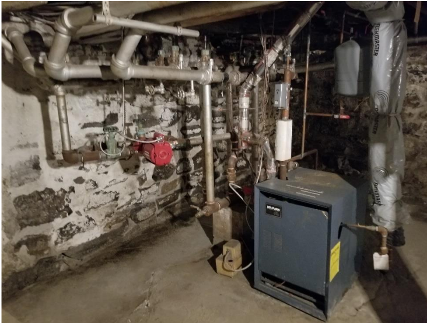
Photo 1: Typical electric boiler connected to radiant heating system. No pipe insulation observed.
