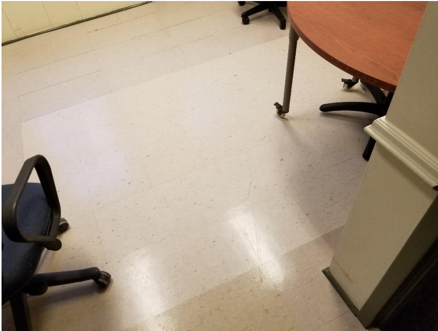
Photo 7: Room 101 which contains all three observed types of non-asbestos VFT.
