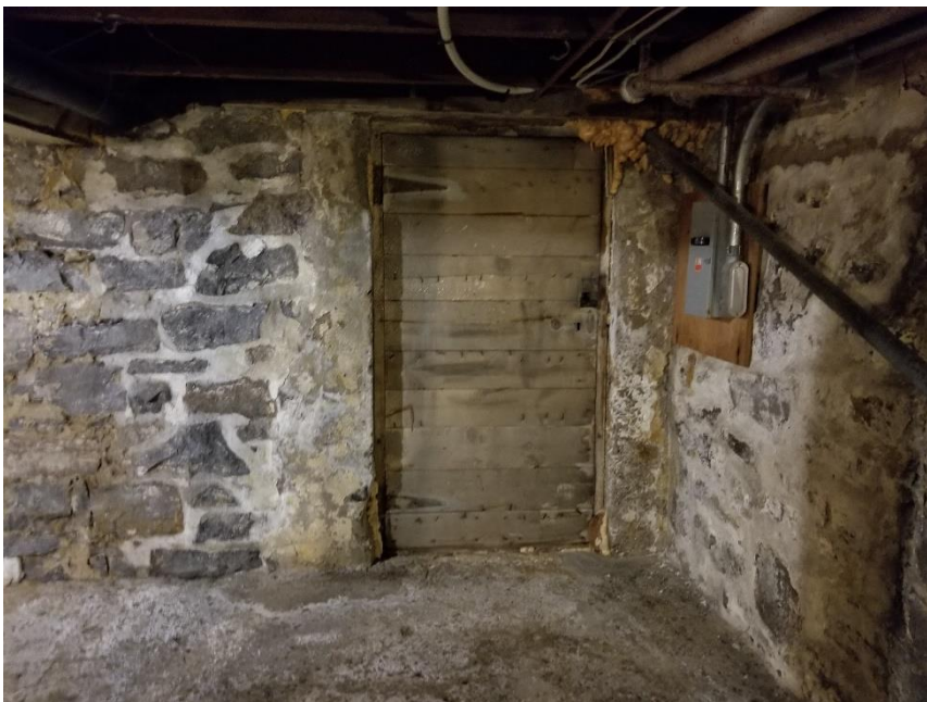
Photo 2: Representative view of the finishes observed throughout the basement level.
