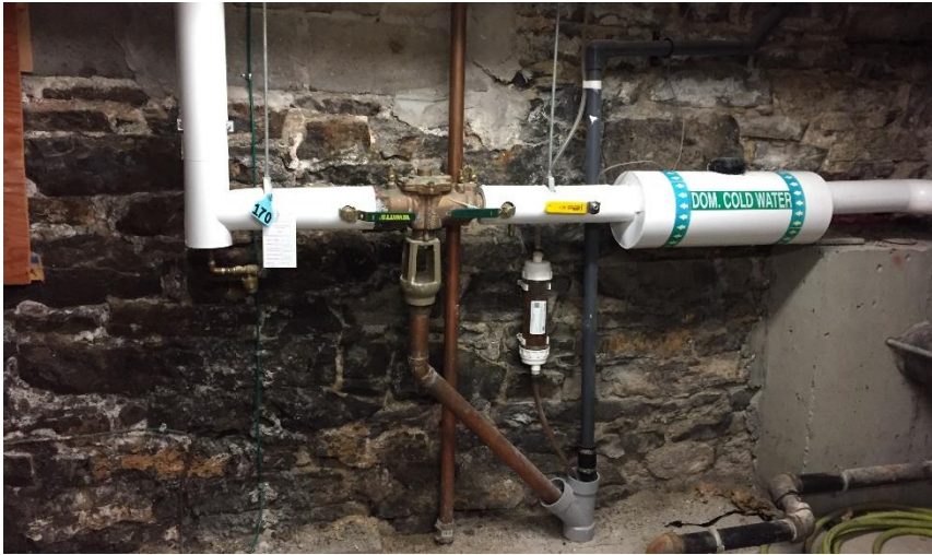
Photo 1: Representative view of the fiberglass insulation observed throughout the subject building.
