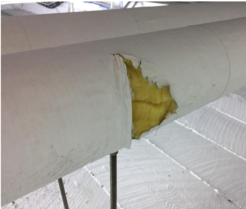
Photo 6: View of fiberglass pipe insulation within the Basement
