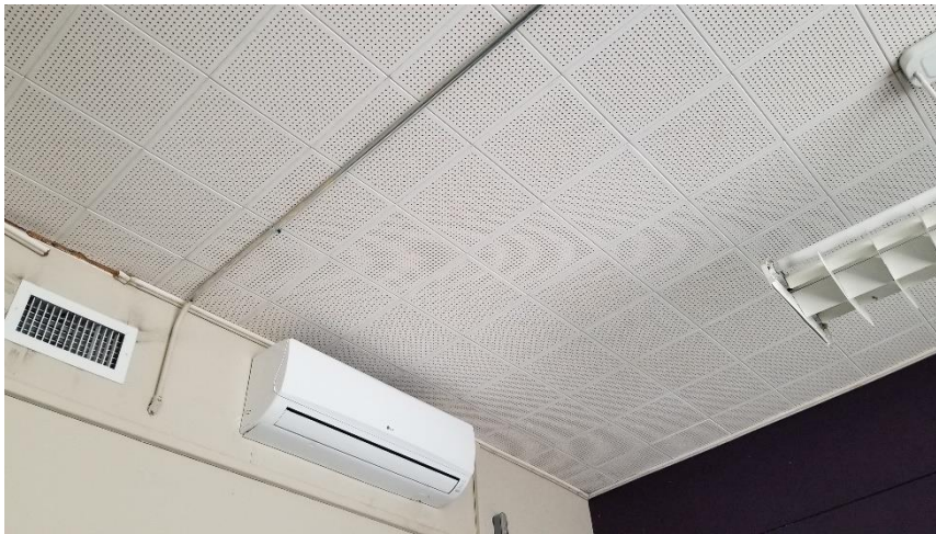
Photo 7: View of the non-asbestos acoustic stick-on ceiling tiles observed in Room 113.
