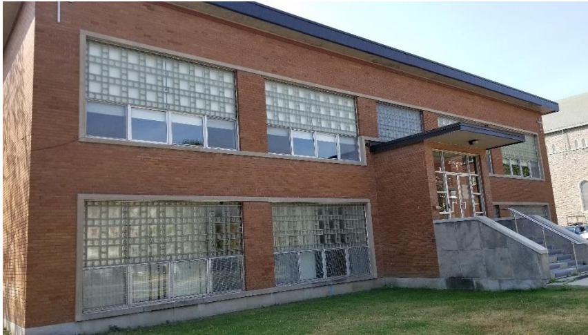
Photo 1: Representative view of the subject building located at 200 Willbrod Avenue.
