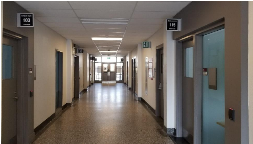
Photo 2: Representative view of the Level 1 main corridor area finishes. No asbestos containing materials were identified in this general area.
