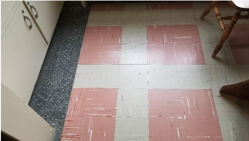
Photo 19: View of the asbestos-containing VFT 9"x9" - Pink & Beige observed in good condition in Room 015A.
