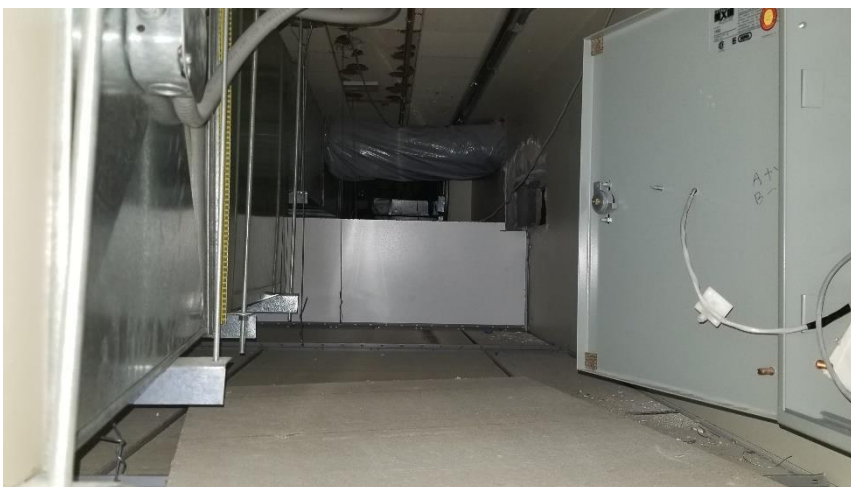
Photo 12: View of the ceiling space above the suspended ceiling tiles observed in the Level 0 corridor. Non-asbestos stick on ceiling tiles and mastic (Dark Brown) were visible.
