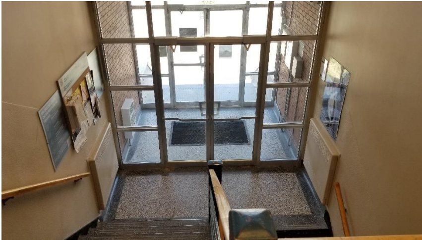
Photo 10: Representative view of the stairwell and vestibule area of the subject building.
