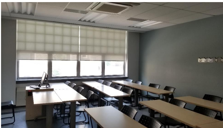
Photo 3: Representative view of Room 102 interior finishes, which were observed to be newly renovated. No asbestos materials are suspected to be present.
