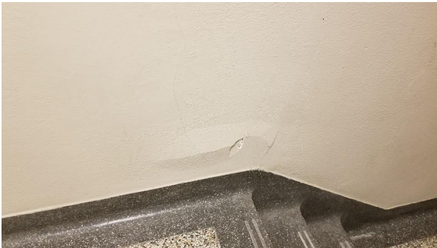
Photo 20: View of the non-asbestos wall plaster observed throughout the subject building.
