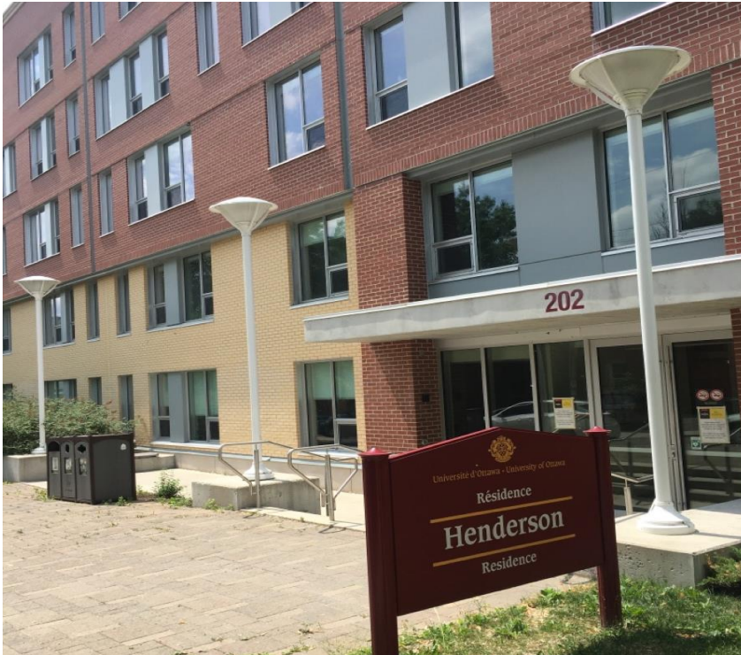
Photo 1: View of building located at 202 Henderson Avenue in Ottawa.
