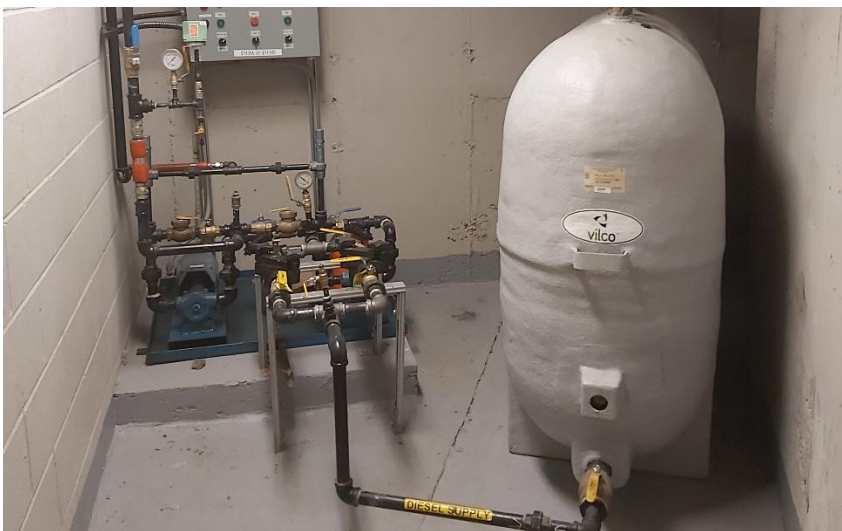
Photo 3: View of the diesel tank identified in Room 01.
