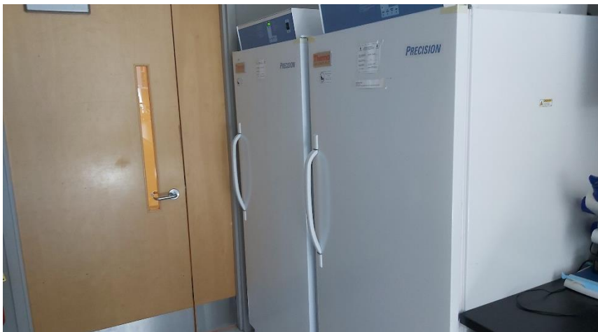
Photo 8: Representative view of the equipment containing ODS's observed throughout the subject building.
