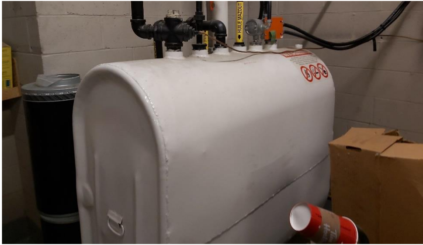
Photo 4: View of the diesel tank identified in Room 508.
