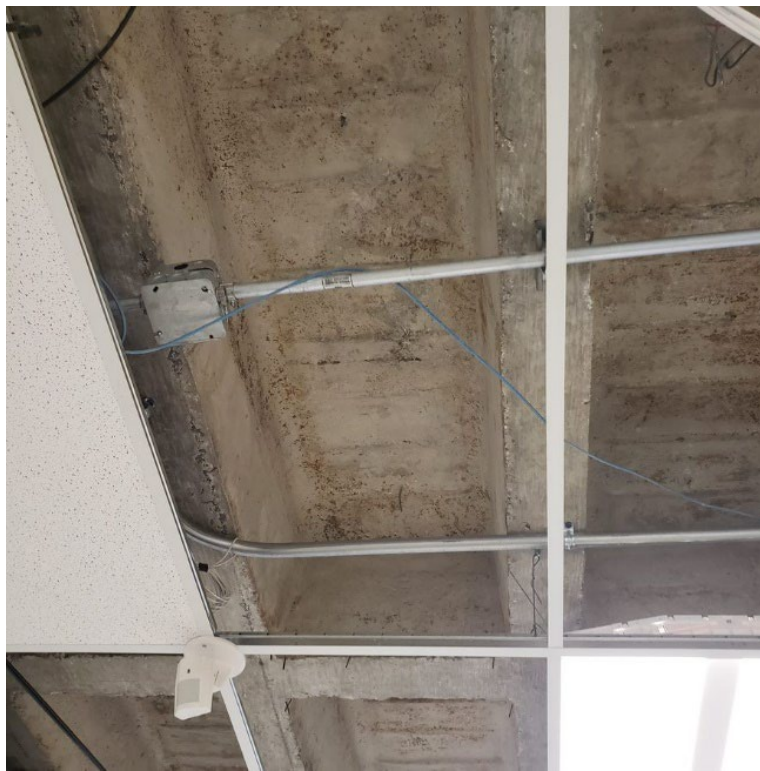
Photo 1. Example of bare concrete ceiling.
