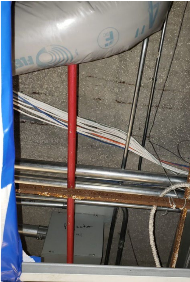
Photo 6. View of minimal overspray on concrete deck.
