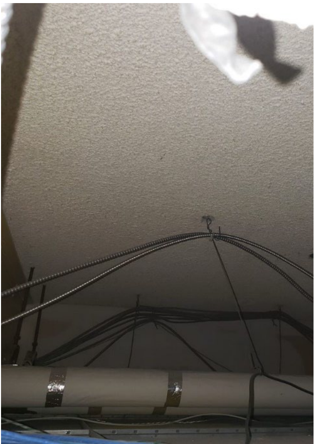
Photo 2. Example of cementitious overspray observed in good condition.
