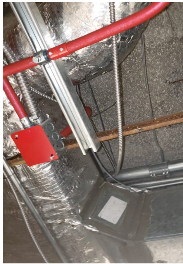
Photo 7. View of minimal overspray on concrete deck.
