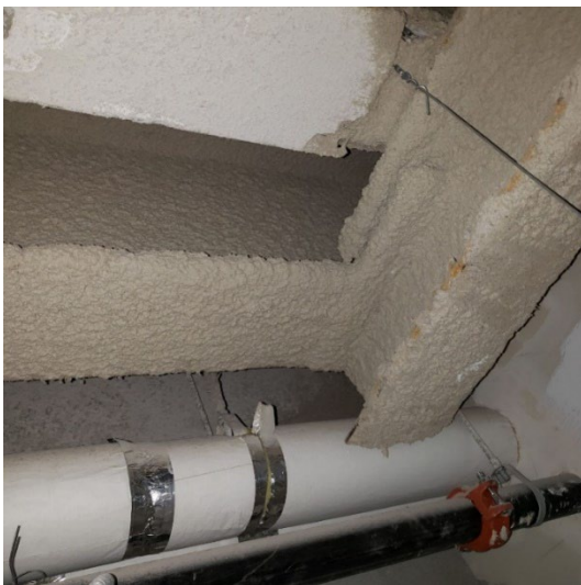
Photo 6. Example of non-ACM beige sprayed fireproofing observed on the 1 st floor.
