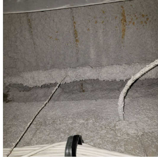
Photo 5. Example of non-ACM grey sprayed fireproofing observed on the 5 th floor.
