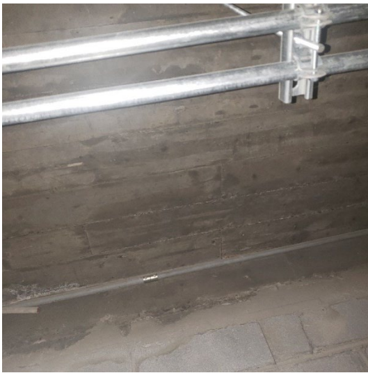
Photo 1. Example of bare concrete ceiling observed on the 6 th floor.
