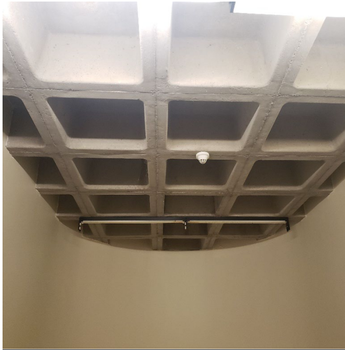
Photo 1. Example of bare concrete ceiling.
