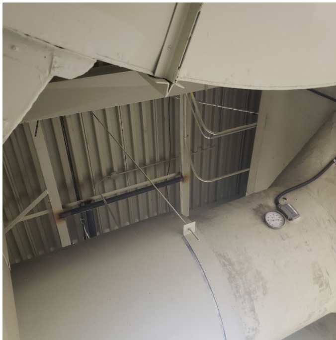
Photo 2. Example of corrugated metal ceiling.
