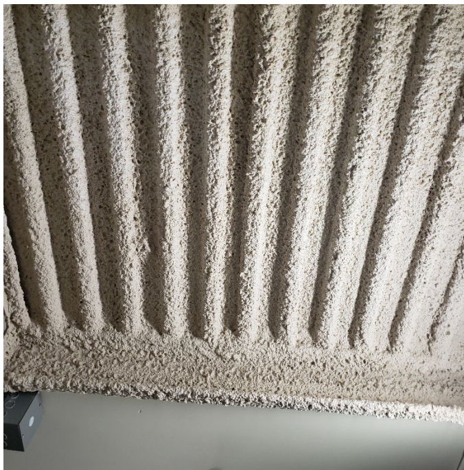
Photo 5. Example of sprayed fireproofing within room 0042B.
