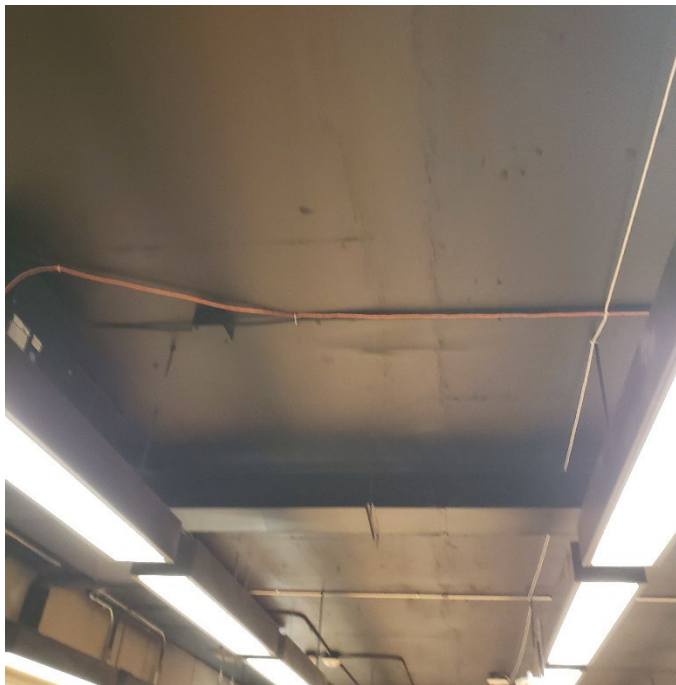
Photo 1. Example of bare concrete ceiling.
