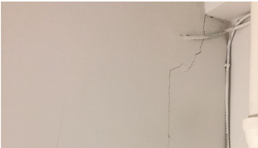
Photo 8: View of the asbestos-containing plaster observed in fair condition in Room 004.
