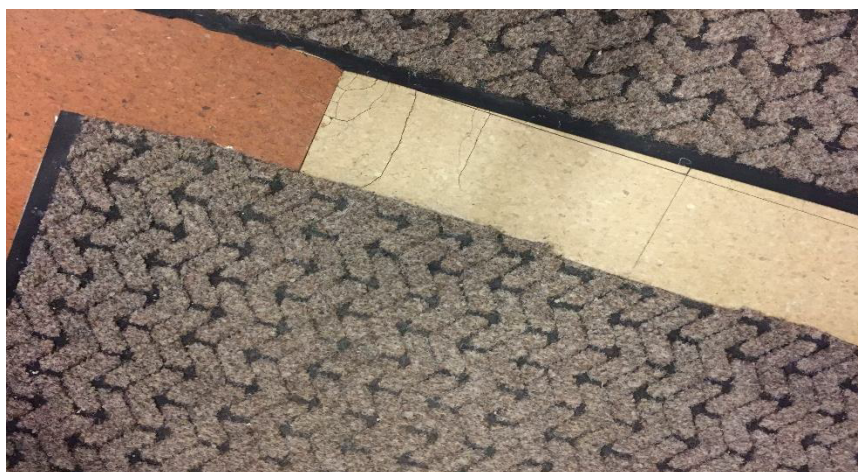
Photo 2: View of non-asbestos-containing vinyl floor tiles observed throughout the subject building.
