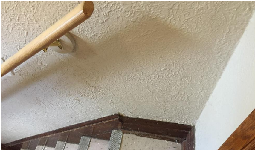
Photo 5: View of the non-asbestos containing wall texture coat observed in Room 10.
