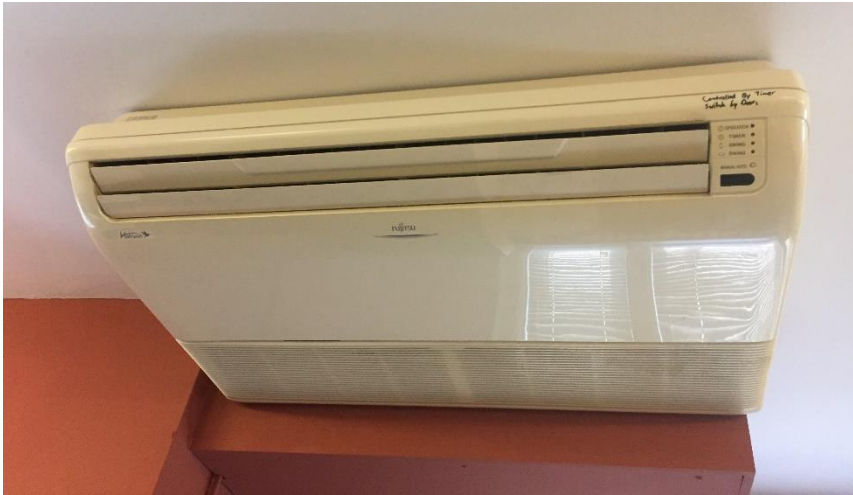
Photo 4: Representative view of equipment observed to contain ODSs throughout the subject building.
