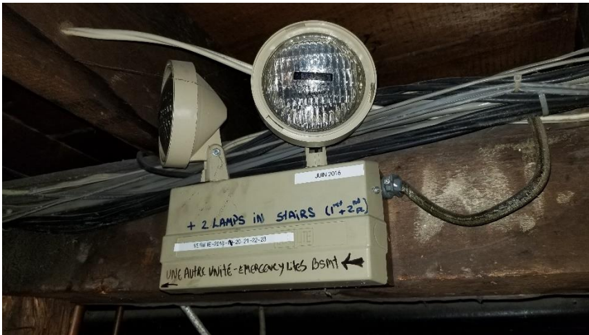
Photo 8: View of the lead-containing battery packs identified in Room B5.
