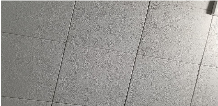
Photo 4: View of non-asbestos ceiling tiles (1' x 1') observed in Room 102.
