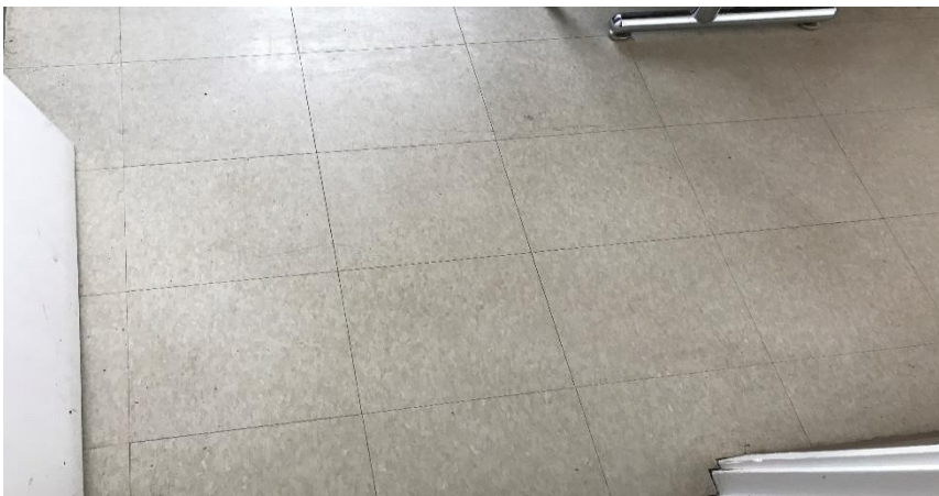
Photo 5: View of asbestos containing 12"x12" vinyl floor tile in Room 201
