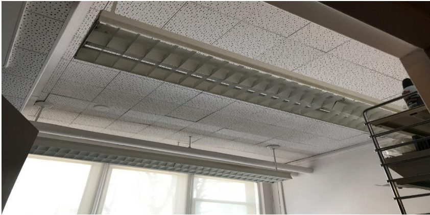
Photo 1: View of non-asbestos ceiling tile (1'x1') in Room 101.
