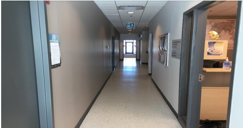
Photo 1: View of typical finishes observed at the building located at 600 Peter Morand Crescent.
