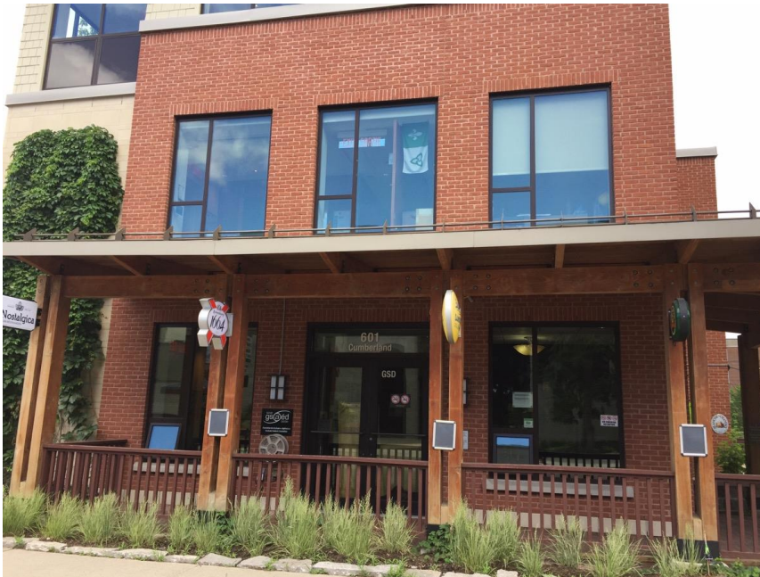
Photo 1: View of the exterior of the building
