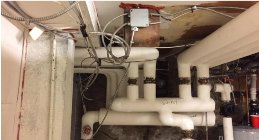
Photo 9: View of the fiberglass insulation observed in Room 005.
