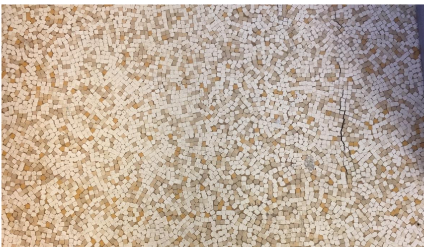
Photo 3: View of the asbestos-containing vinyl sheet flooring (White with Brown Squares) observed in Room 103.
