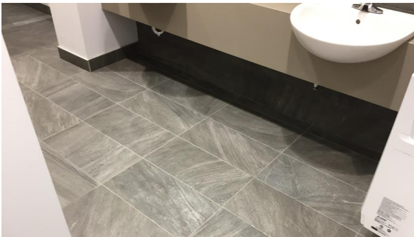
Photo 6: Typical view of ceramic floor tile grout observed throughout the subject building suspected of containing asbestos.
