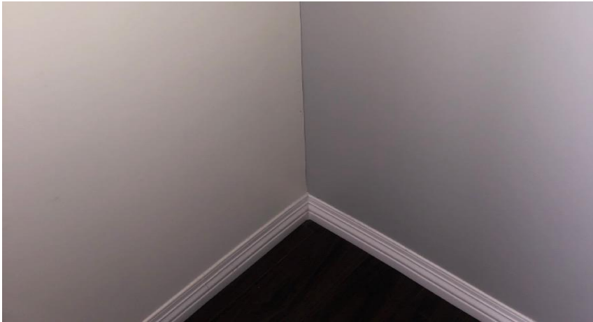
Photo 4: Typical view of light grey wall paint and white trim paint suspected of containing lead.
