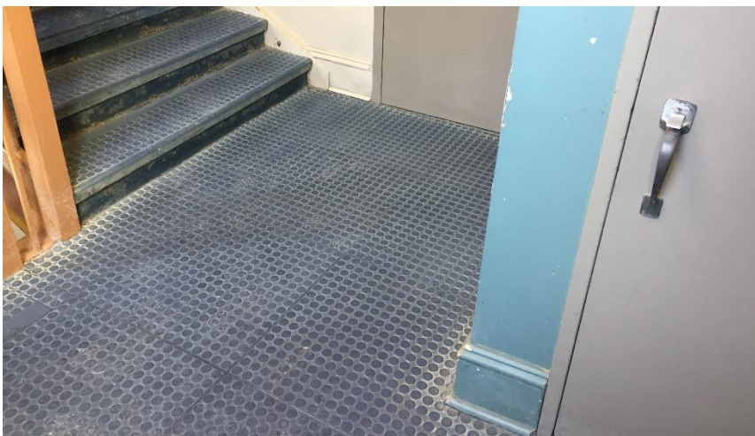
Photo 6: View of non-asbestos containing vinyl sheet flooring in Room 101.
