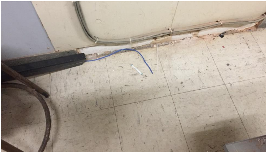
Photo 5: View of asbestos-containing vinyl floor tiles in Room 017.
