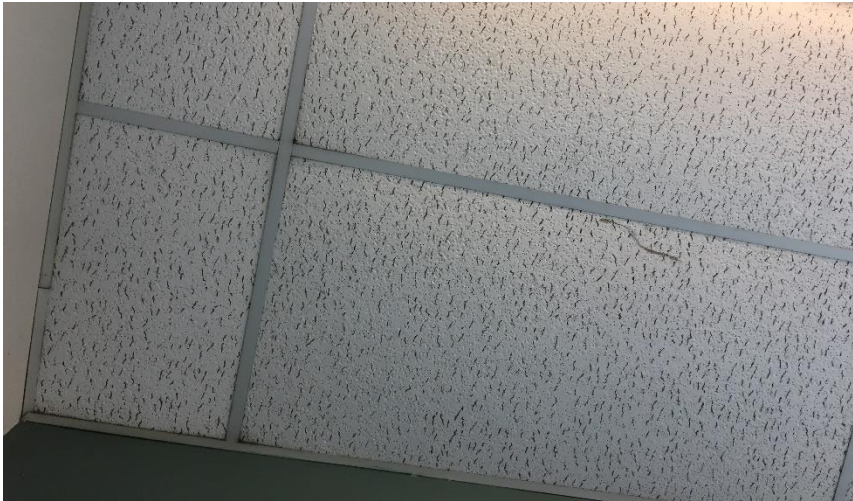
Photo 10: View of non-asbestos containing suspended ceiling tiles in Room 300.
