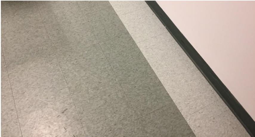
Photo 1: View of non-asbestos containing vinyl floor tile (12" x 12" -green) observed in Room 309.
