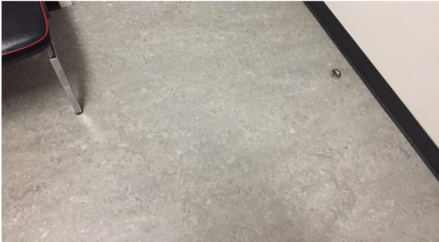
Photo 7: View of non-asbestos containing vinyl sheet flooring in Room 302.
