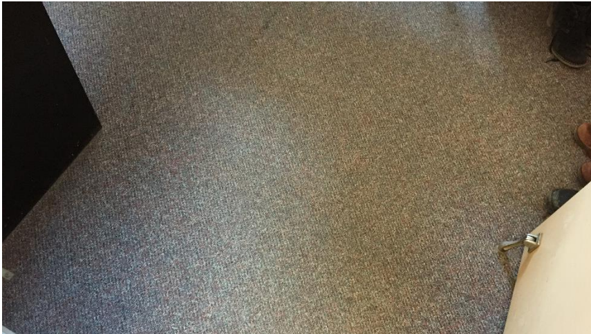
Photo 14: View of non-asbestos containing carpet mastic in Room 209.
