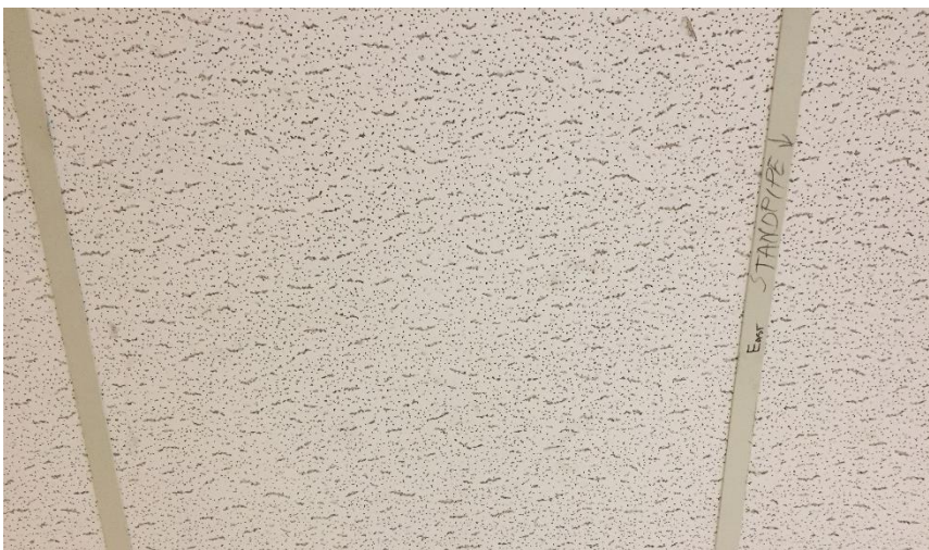
Photo 9: View of non-asbestos containing suspended ceiling tiles in Room 001.
