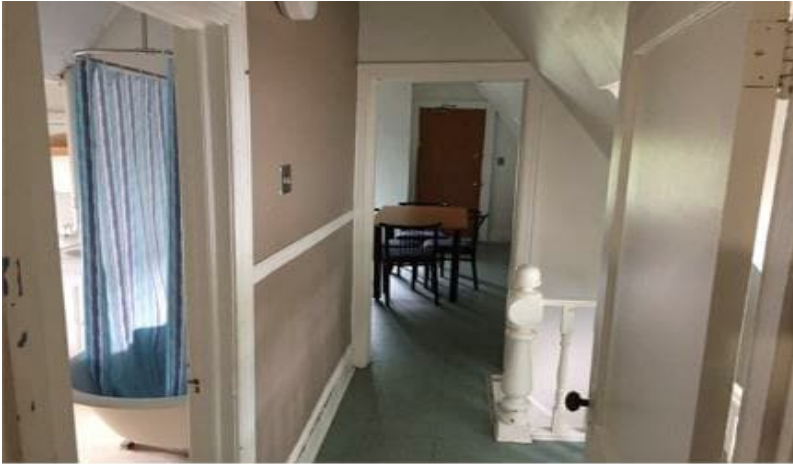
Photo 1: View of typical finishes observed at the building located at 116 Henderson Avenue.
