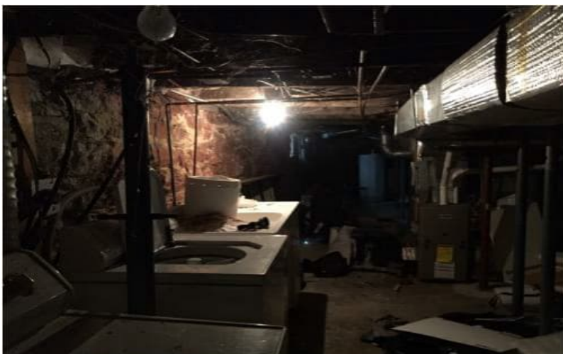
Photo 3: View of typical finishes observed at the building located at 122 Henderson Avenue.
