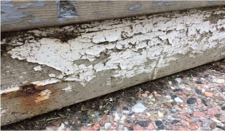
Photo 7: View of lead-containing white paint observed to be in poor condition on the front deck.
