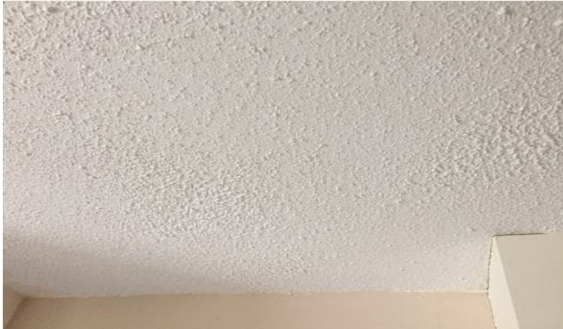
Photo 4: View of non-asbestos-containing ceiling texture coat observed in the 2nd-floor bathroom.
