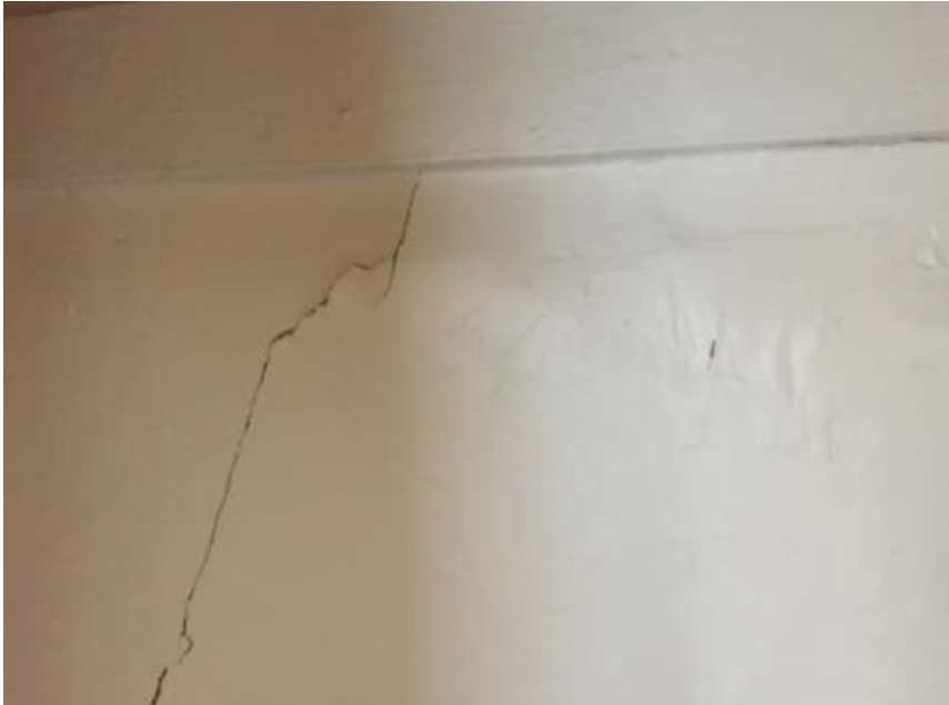
Photo 7: View of asbestos-containing plaster observed in poor condition in Room 209A of 15 Stewart Street.
