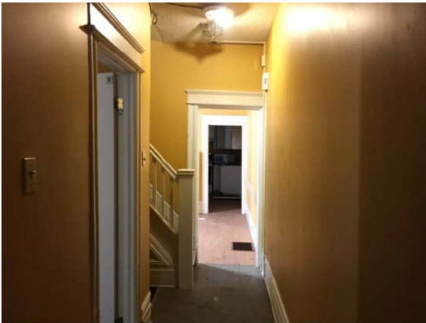
Photo 2: Representative view of the interior finishes observed at 15 Stewart Street.
