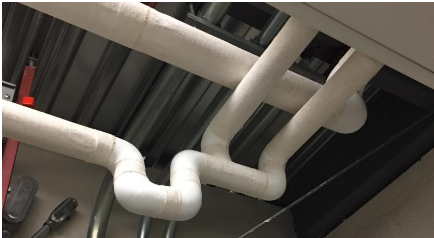
Photo 4: Representative view of the non-asbestos-containing mechanical insulation observed throughout the subject building.
