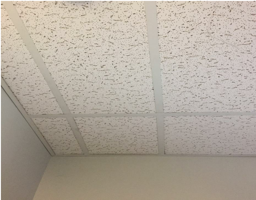
Photo 2: Typical view of non-asbestos-containing suspended ceiling tiles with large fissures observed within Room 111.
