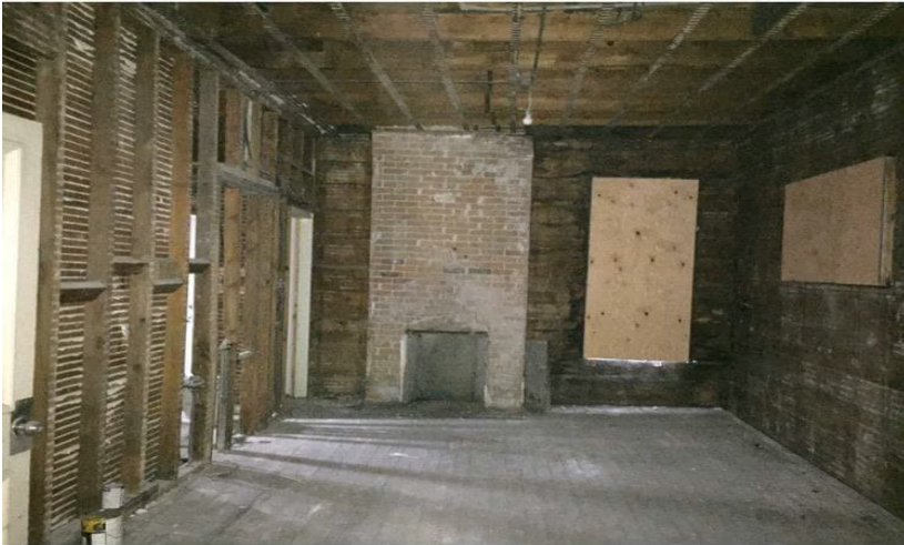
Photo 2: Typical view of building finishes observed within the subject building.
