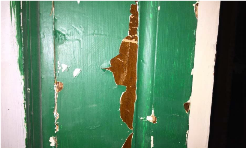
Photo 4: View of green lead-containing paint observed to be damaged near the stairs to the 2 nd floor.
