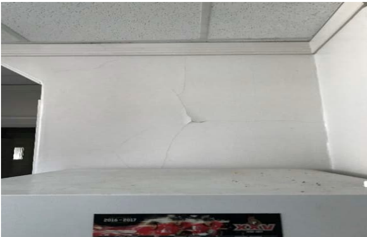
Photo 2: View of lead-containing white paint observed to be in fair condition in the foyer of the subject building.
