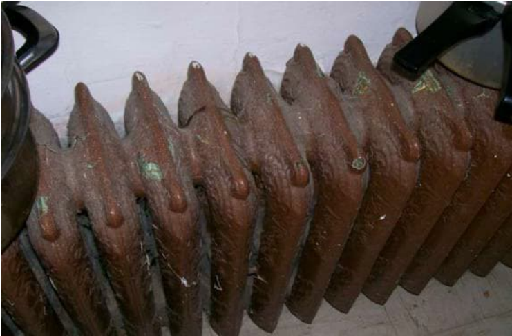
Photo 4: View of lead-containing brown paint observed to be in good condition in the dining room of the subject building.
