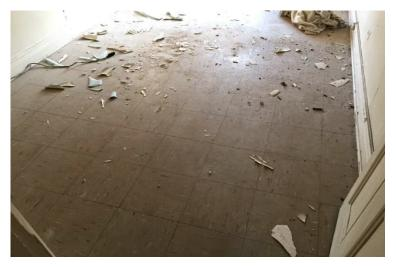
Photo 3: View of asbestoscontaining vinyl floor tiles (12"x12"-grey with white and black streaks) observed in Room 302.
