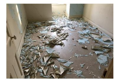
Photo 4: View lead-containing light blue paint was observed to be in poor condition in Room 301.
