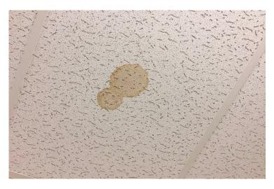
Photo 6: View of waterdamaged suspended ceiling tile observed in Room 101.
