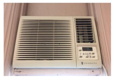
**Photo 5:** Typical view of ODS containing airconditioning unit.
