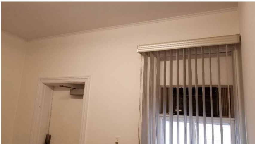
Photo 6: Typical wall and ceiling plaster finished observed in Room 110.
