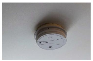
**Photo 6:** Typical view of smoke detectors containing radioactive materials.
