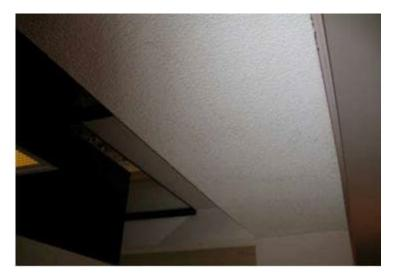
Photo 4: View of asbestoscontaining ceiling texture coat observed in Room 100A.
