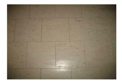
Photo 3: View of asbestoscontaining vinyl floor tile observed in Room B15B.
