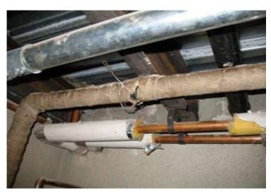
Photo 2: View of asbestoscontaining thermal wrap observed in Room B6B.
