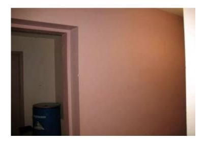
Photo 5: View of dark purple lead-containing paint observed on the wall in Room B1.
