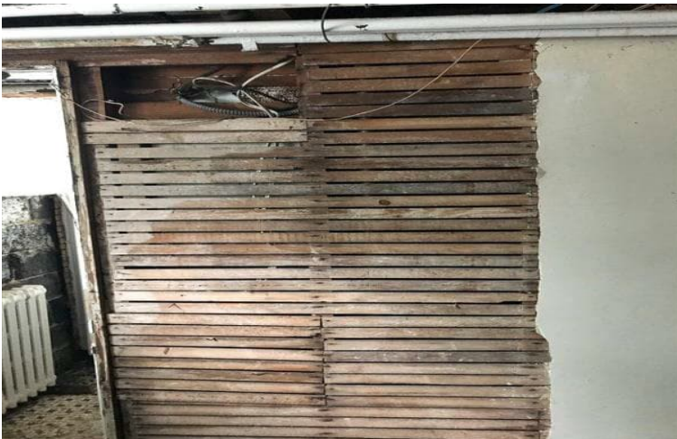
Photo 2: View of typical finishes observed at the building located at 599 King Edward Avenue.
