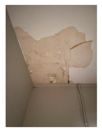
Photo 3: View of water damaged ceiling observed within Apartment 2 of the subject building.
