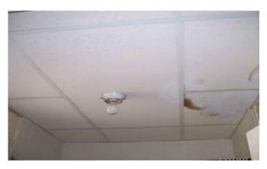
Photo 2: View of water damaged ceiling tiles observed in the bathroom (Room 106) on the 1st floor of the subject building.
