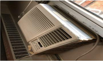
**Photo 4:** Typical view of ODS containing airconditioning unit.
