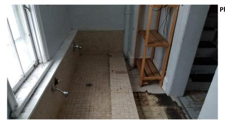
Photo 2: View of non-asbestos vinyl sheet flooring underneath vinyl floor tiles in Room 105.
