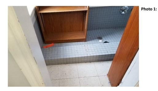
View of non-asbestos vinyl floor tiles (12" x 12") and ceramic floor tile grout suspected of containing asbestos in Room 205.
