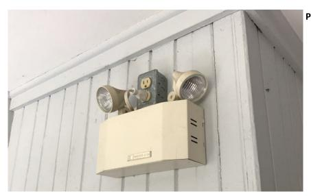
Photo 5: View of leadcontaining batteries observed in Room 100.
