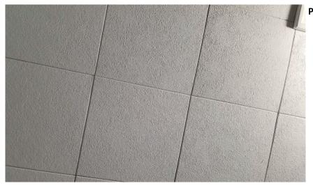
Photo 4: View of non-asbestos ceiling tiles (1' x 1') observed in Room 102.
