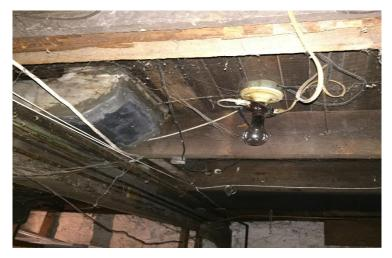
Photo 8: View of asbestoscontaining duct insulation observed in Room 01.
