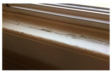
Photo 11: View of low level lead white wall paint observed to be in poor condition in Room 202.
