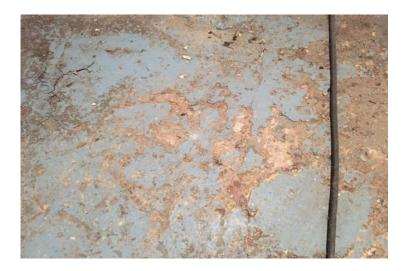
Photo 10: View of leadcontaining blue floor paint observed to be in poor condition in Room 01.
