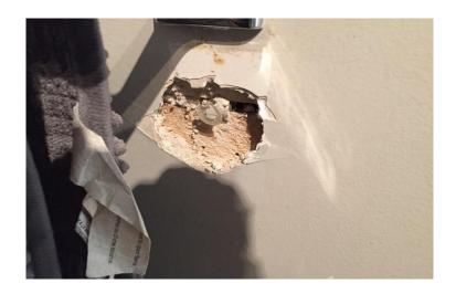
Photo 7: View of asbestoscontaining plaster in Room 204 observed to be in poor condition.
