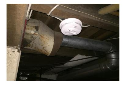
**Photo 12:** Typical view of smoke detectors containing radioactive materials.
