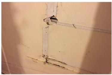
Photo 6: View of asbestoscontaining plaster in Room 201 observed to be in poor condition.
