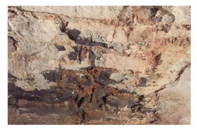
Photo 9: View of asbestoscontaining wall texture coat observed to be in poor condition in Room 01.
