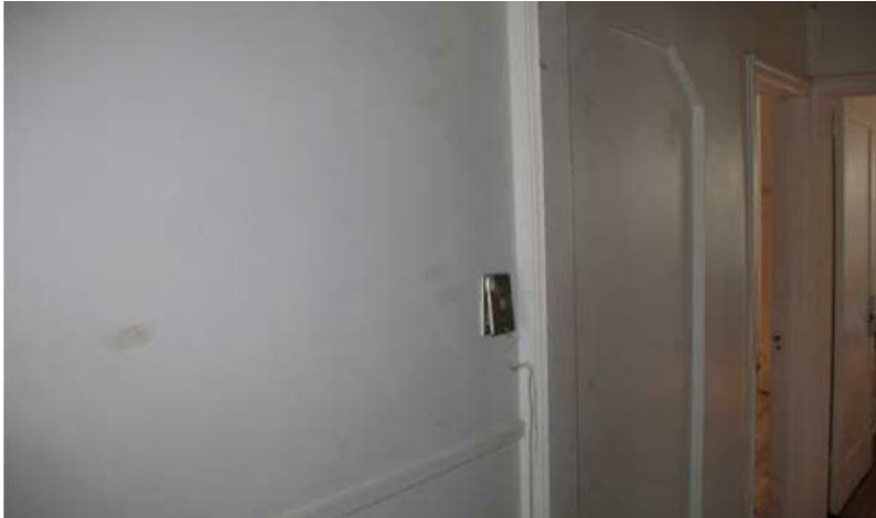
Photo 1: View of typical finishes observed at 80 Templeton Street.
