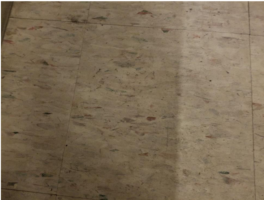
Photo 4: View on non-asbestos containing vinyl floor tiles (12"x12"-Beige w/ Brown Flakes)
