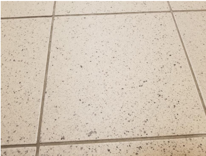
Photo 6: View on non-asbestos containing vinyl floor tiles (12"x12"-Grey w/ Dark Flakes)
