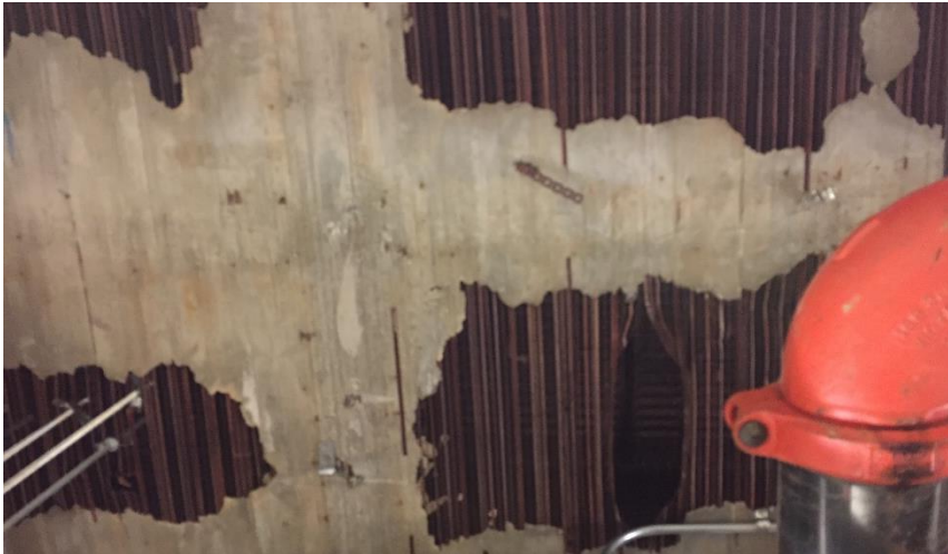
Photo 7: View of the non-asbestos containing ceiling plaster observed in Room 005.
