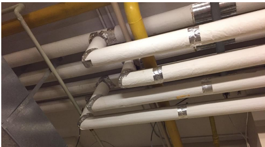
Photo 10: Representative view of the non-asbestos containing mechanical insulation observed in Room 0015.
