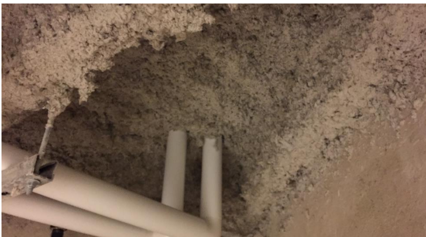
Photo 9: View of the non-asbestos containing sprayed fireproofing (Grey) observed in Room 07.
