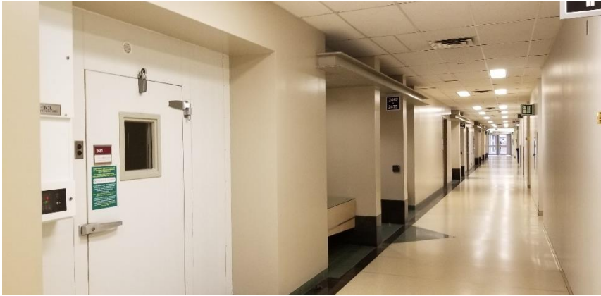
Photo 22: Representative view of the second level common area finishes.
