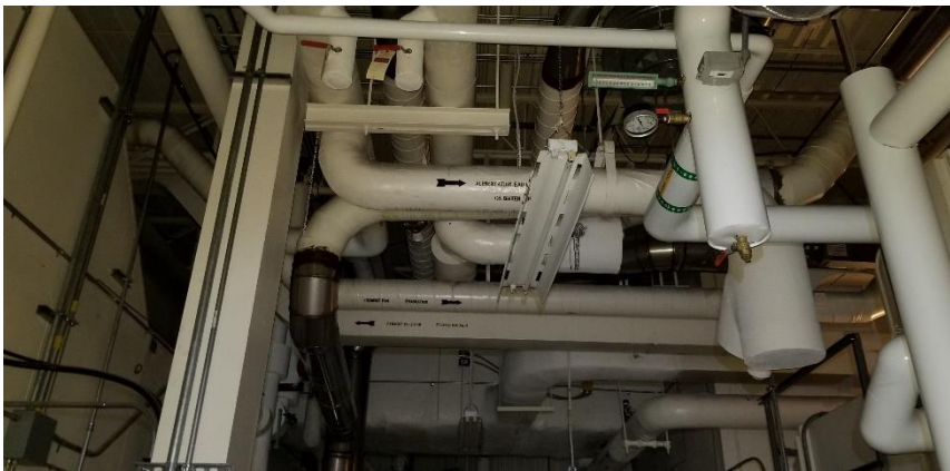
Photo 38: Representative view of the fiberglass mechanical insulation observed in Room 5004.
