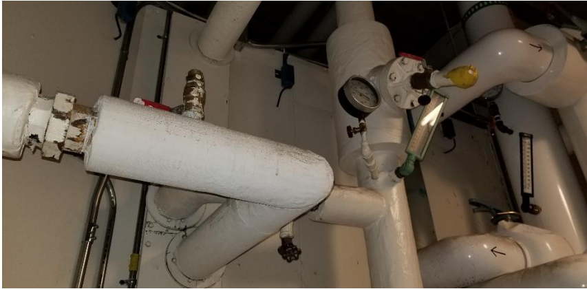
Photo 40: Representative view of the fiberglass mechanical insulation observed in Room 5002.
