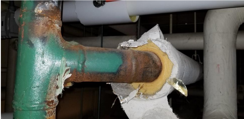
Photo 10: Representative view of the fiberglass insulation observed in Room 1138.
