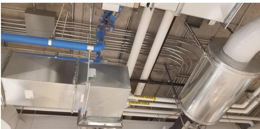
Photo 18: Representative view of the fiberglass insulation observed in Room 1500J.
