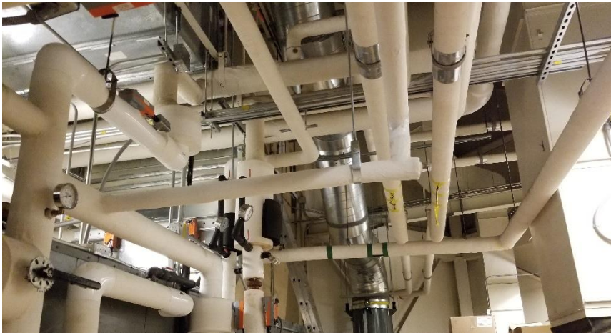
Photo 34: Representative view of the fiberglass mechanical insulation observed in Room 3003B.
