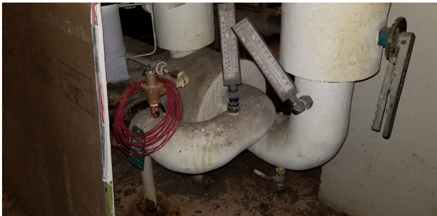
Photo 8: Representative view of the non-asbestos pipe elbow/fitting insulation observed in Room 1138.
