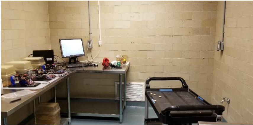
Photo 19: Representative view of the room finishes observed in Room 1201.
