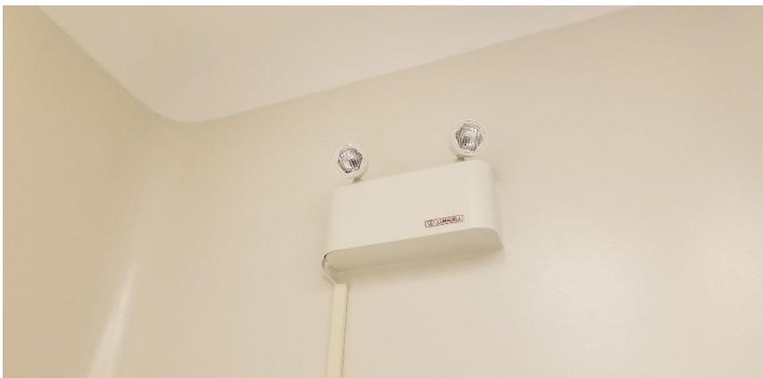
Photo 21: Representative view of the lead battery packs observed in Rooms 1326A & 1326C.
