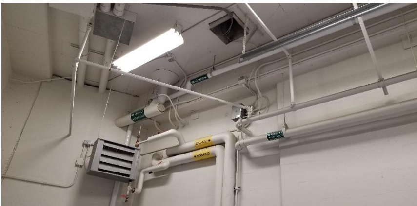
Photo 15: Representative view of the fiberglass insulation observed in Room 1506.
