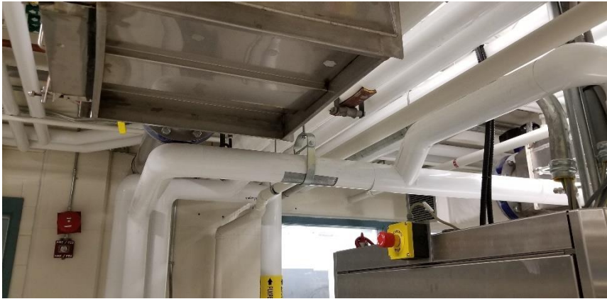
Photo 4: Representative view of the fiberglass insulation observed in Room 0516A/B.
