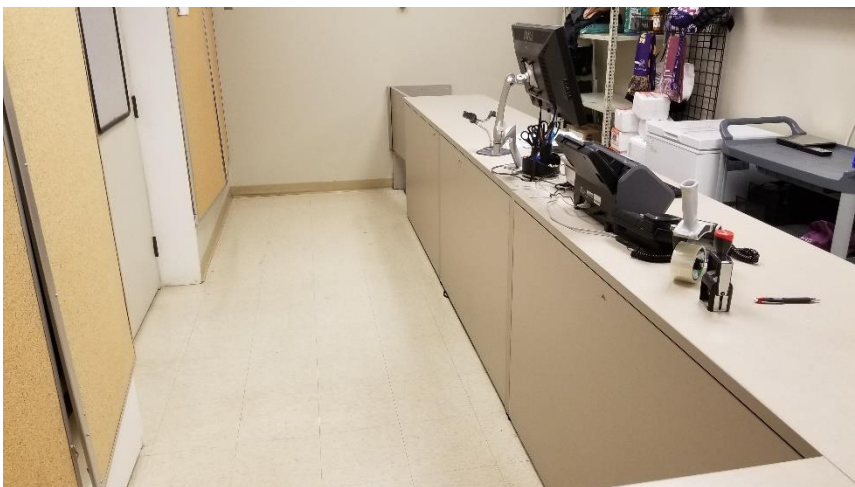
Photo 27: View of the non-asbestos VFT (12"x12" Beige w/ Brown Flakes) observed in Room 1129A.
