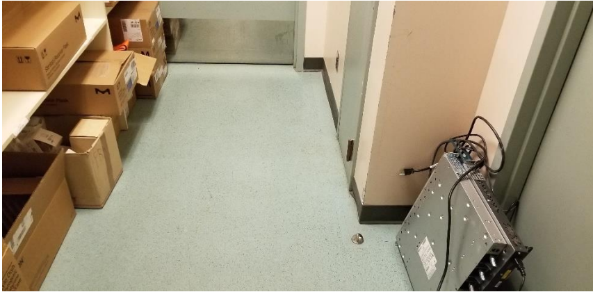
Photo 28: View of the non-asbestos VFT (12"x12" - Blue w/ Black Dots ) observed in Room 2482.
