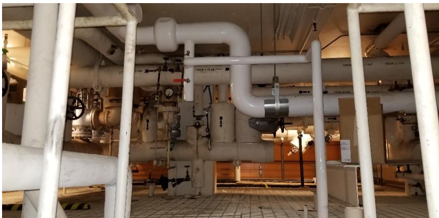
Photo 9: Representative view of the fiberglass insulation observed in Room 1138.
