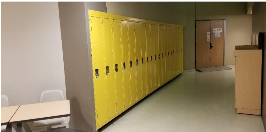
Photo 29: Representative view of the yellow lead paint observed on lockers throughout the subject building.
